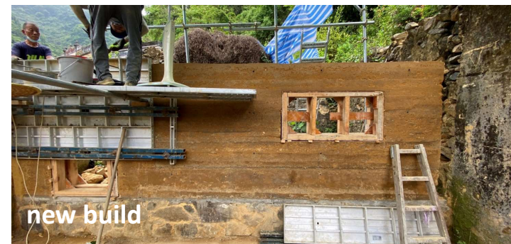
Site visits + demonstrations Lightweight scaffolding, Rammed earth walls
